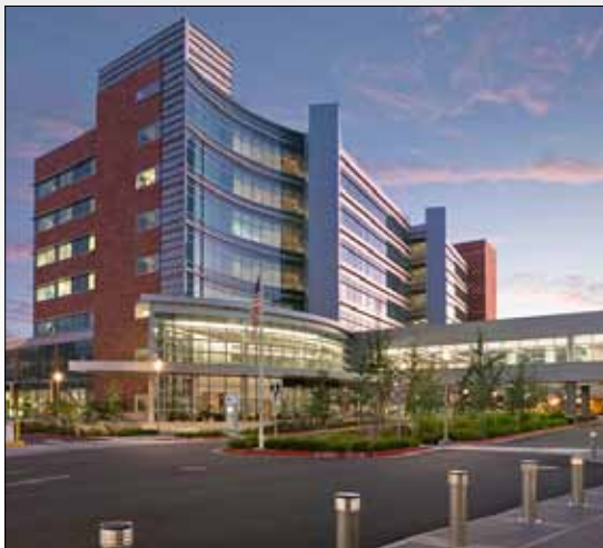
PG LifeLink Isolated Power Installation: Salem Hospital, Salem, OR
