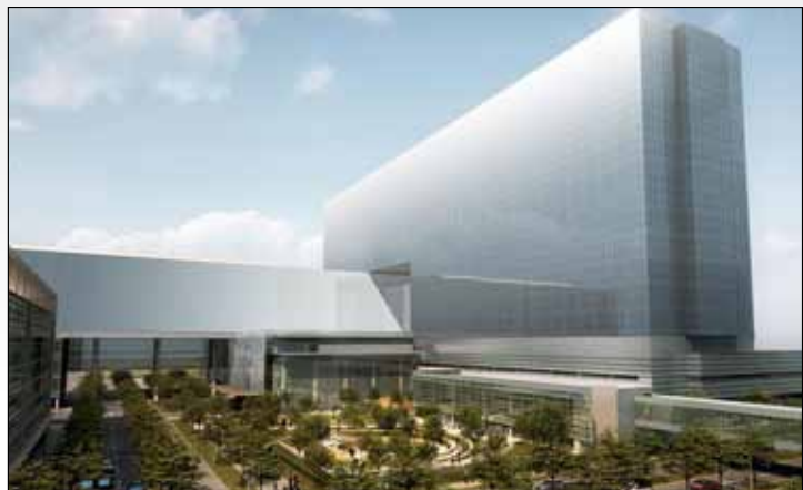
PG LifeLink Isolated Power Installation: Parkland Hospital, Dallas, Texas
