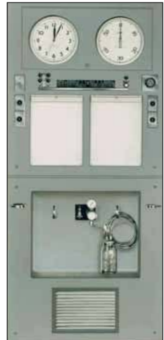
1972 Post Glover Isolated Power Panel
